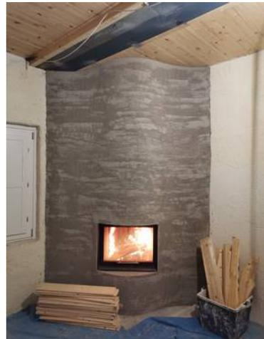
POSA A CALDO DI INTONACO AD ALTA INERZIA TERMICA A BASE DI ARGILLA REFRATTARIA **TERRACCUMULO** (2961 Kg/mc)
